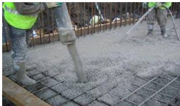
Fig 4: Showing that workability is more and pumping will be easy.
