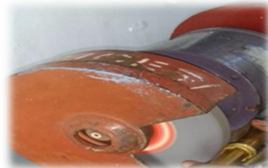
Fig 11. Removing excess material at the weld joint.
