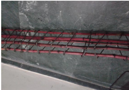
Figure3:- placement of the bamboo
