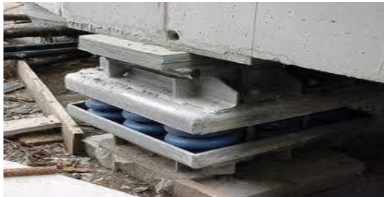
Figure4. Present isolation system
