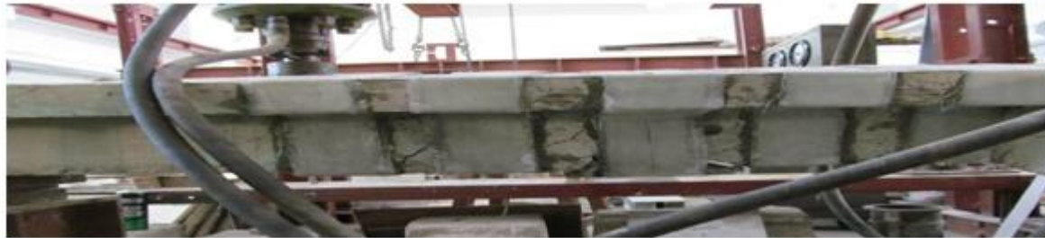
Figure-6 Beams retrofitted with Fully-wrapped GFRP oriented at 90°
