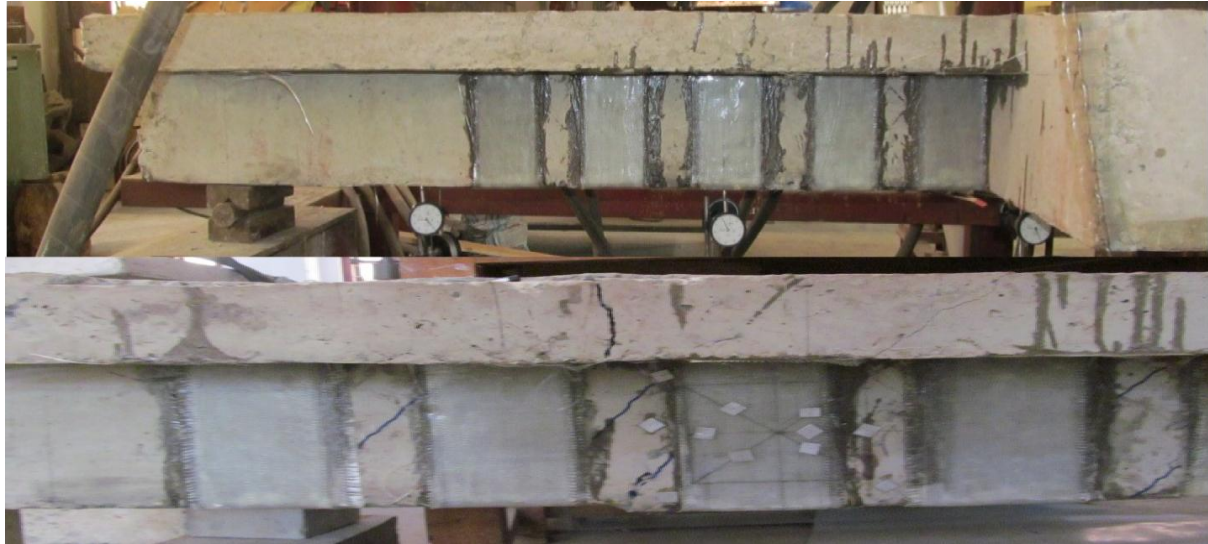
Figure-5 Beams retrofitted with U-wrapped GFRP oriented at 90°
