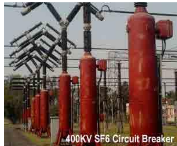
FIG-1 SF 6 CIRCUIT BREAKER
