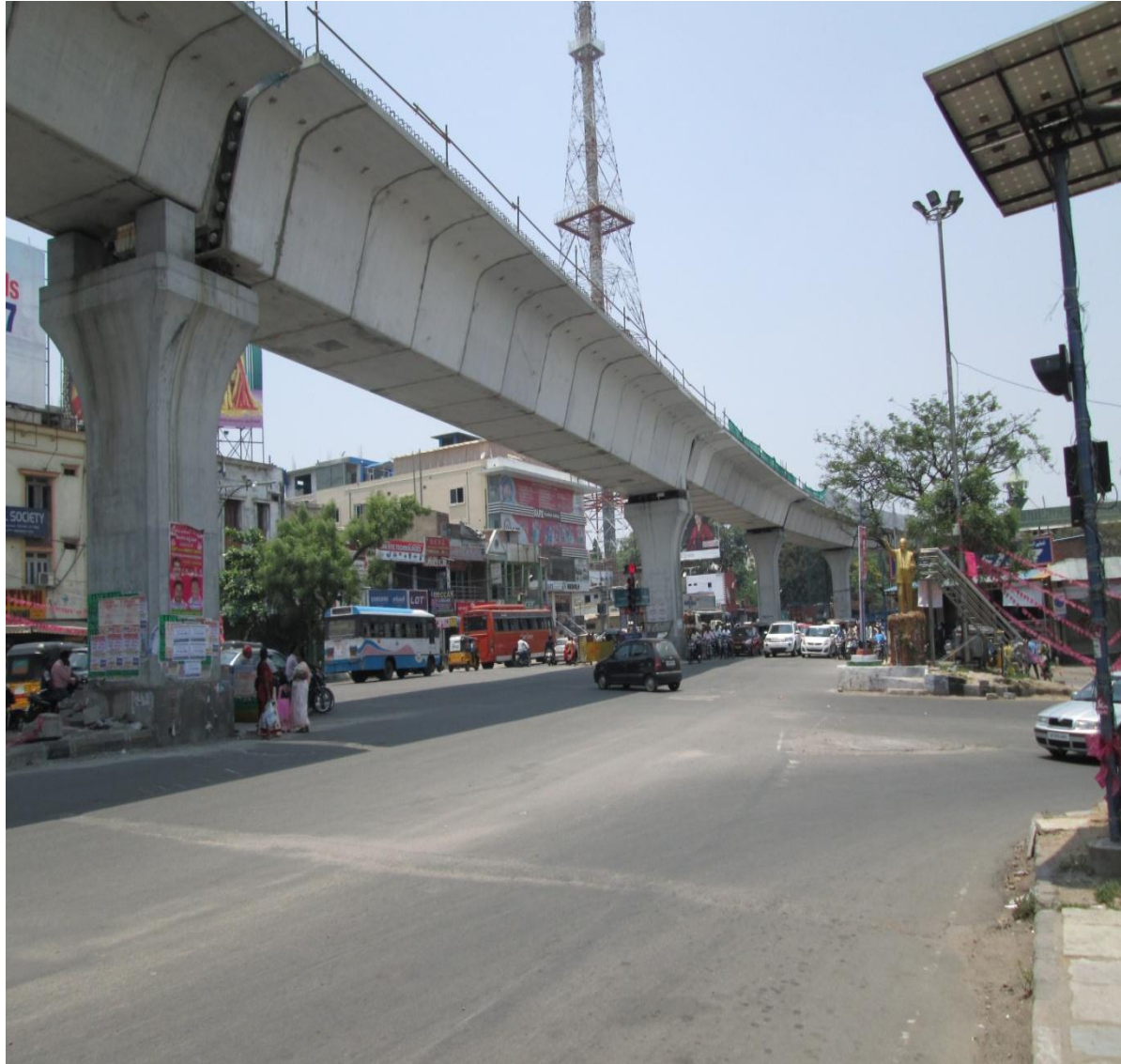
Fig.3.1: T.V tower junction
