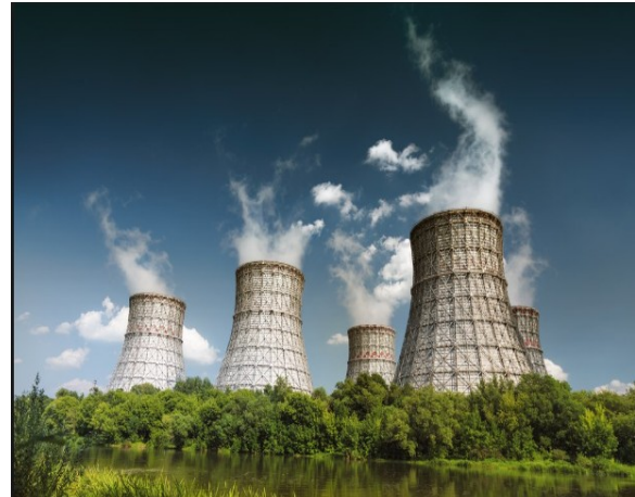
Fig: natural draught cooling towers
