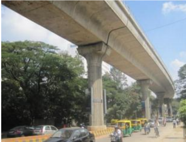
Figure Typical Elevated Metro Bridge
