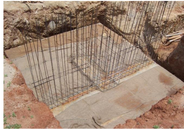
Figure 9.0 Showing the Foundation with partial Shuttering
