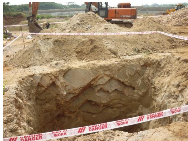
Figure 5.0 showing the Foundation pit showing soft rock at Site
