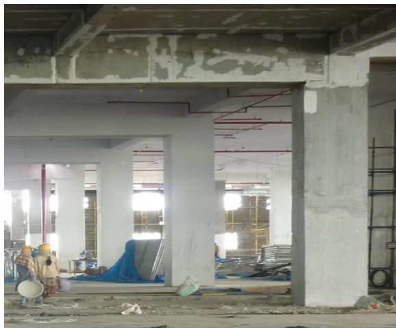
Figure 16.0: Showing the column without Plastering
