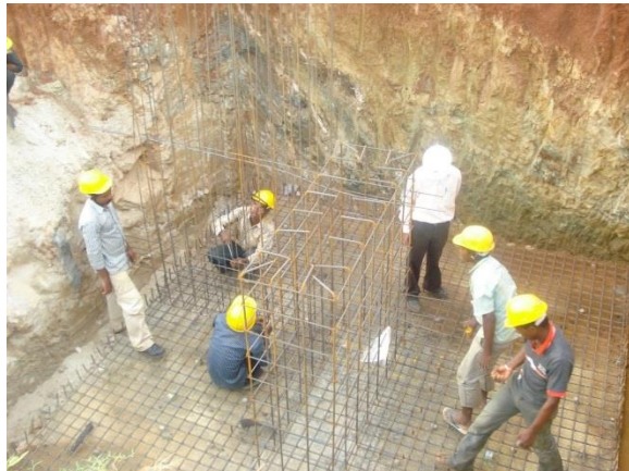
Figure 18.0: Showing the use of Fe500
