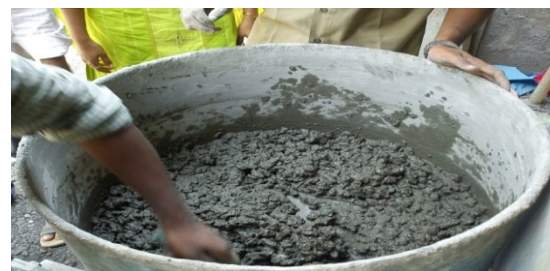
Mixing of concrete
