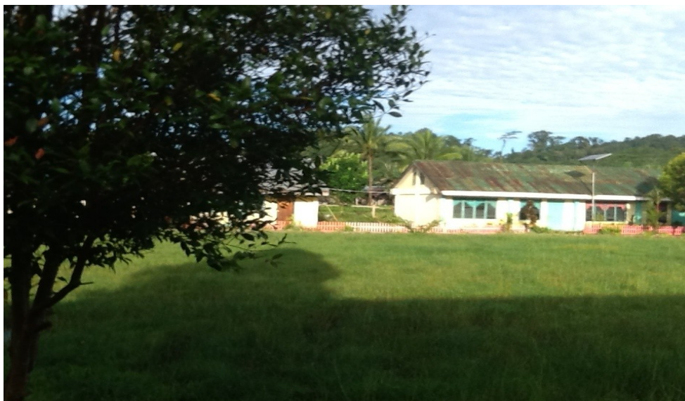
Plate No. 9 A school building of Pakwan Integrated School installed with solar panel, Date taken Feb. 07, 2017(photo courtesy by Rudy Daling)
