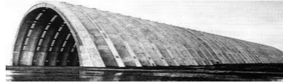
The parabolic-arched airship hangar at Orly Airport in Paris, France
