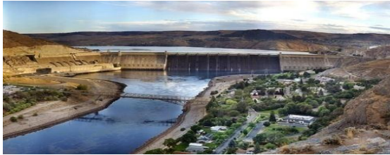
The Grand Coulee Dam
