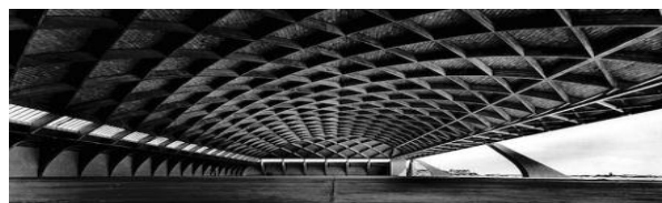
Cast-in-place hangars for the Italian Air Force
