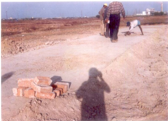
Fig.4 View of compacted surface (soil with 20% FA)
