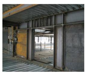
Figure 1: Steel Plate Shear Wall
