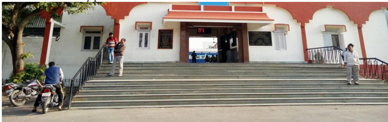
Figure-1 Perspective view of the Railway station where there is no ramp facility
