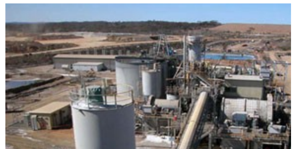
Figure: Attock Cement Pakistan Plant
