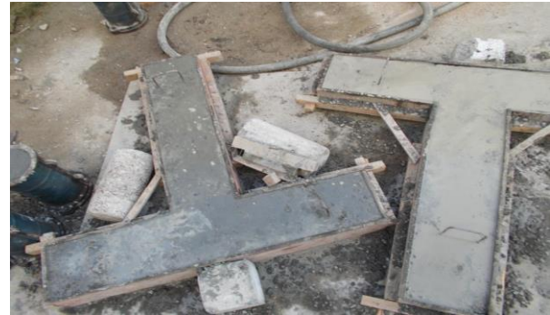
Fig. 2.0 Casting of Beam-Column joint.
