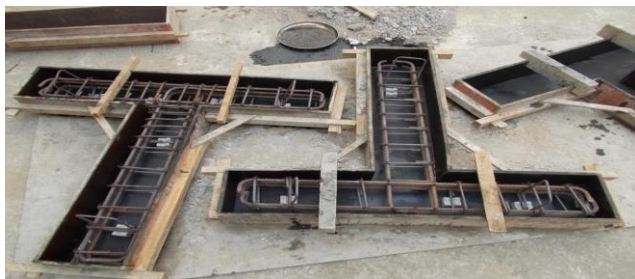
Fig. 1.9 Form work of Beam-Column joint
