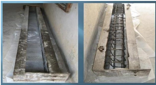
Fig. 3.3 Steel Frame Used For Casting of Beam
