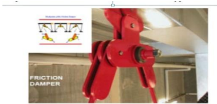
Fig 3:Friction dampers
