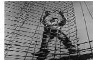
Fig 2. constructing a rebar cage
