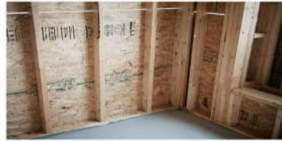
Figure 5 Plywood shear wall
