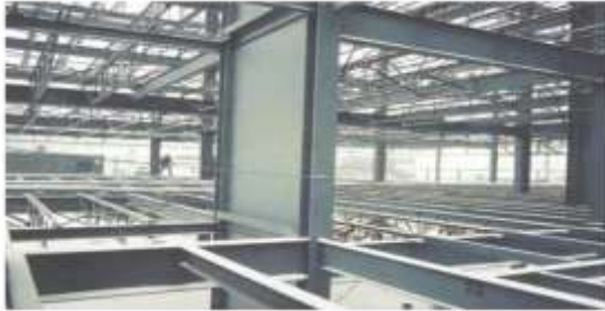
Figure 6 Plate shear wall
