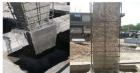
Fig 2. Beam column junction strengthening in basement
