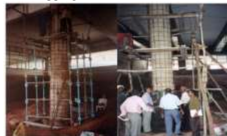
Fig 1. Column jacketing at basement stage
