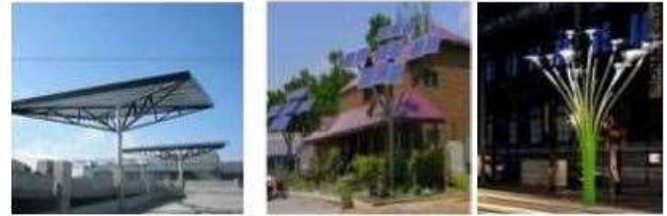
Fig.6. Industrial power House supply Street Light
