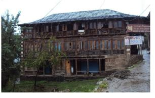
In some constructions tholas can be seen in the upper storey directly above the posts of the verandah which is considered to be a poor construction practice. Thathara houses usually have gable roofs with a slope of about 17 degrees. Over the
