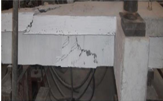
Fig. 4.2 Cracks Pattern in T2C
