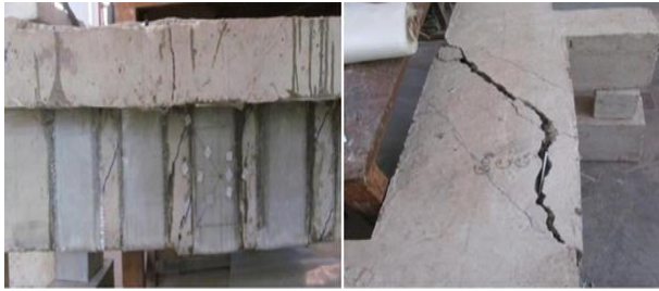
4.4(a) Initial hairline crack
