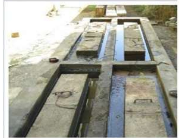
Fig.1 Beam specimens underneath expanded corrosion.
