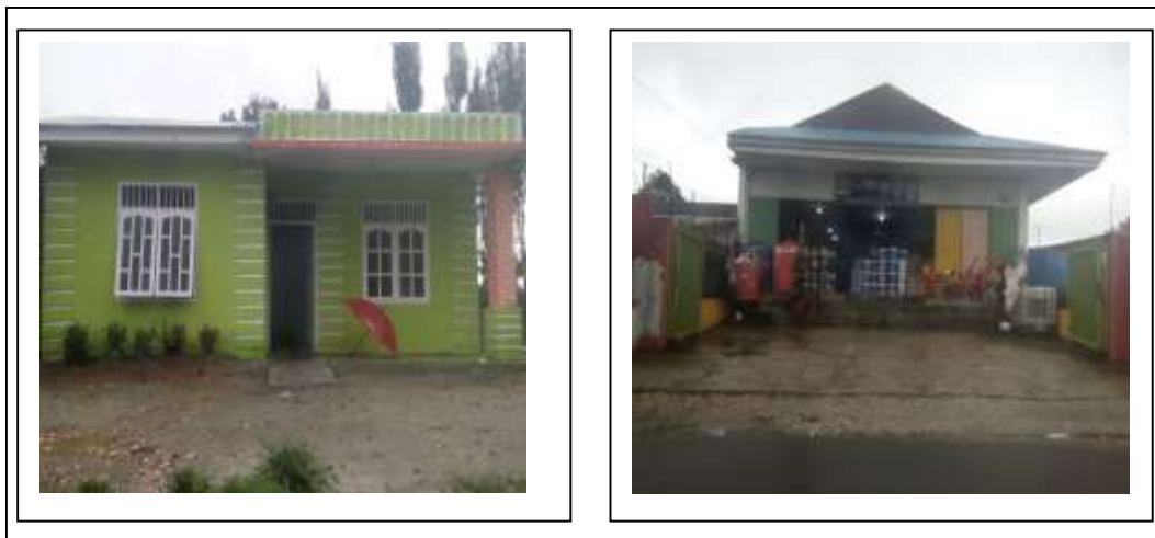
Figure 2. Buildings that violate the road border line
