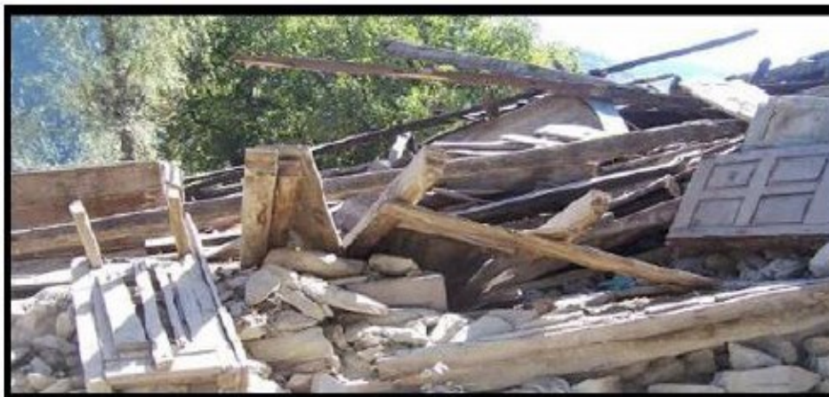
Stage IV of Earthquake. Damage
