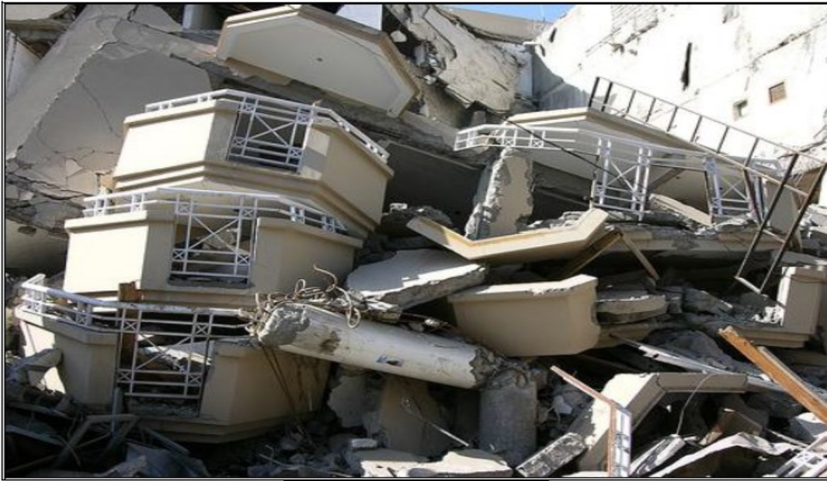
A total collapse of a building
