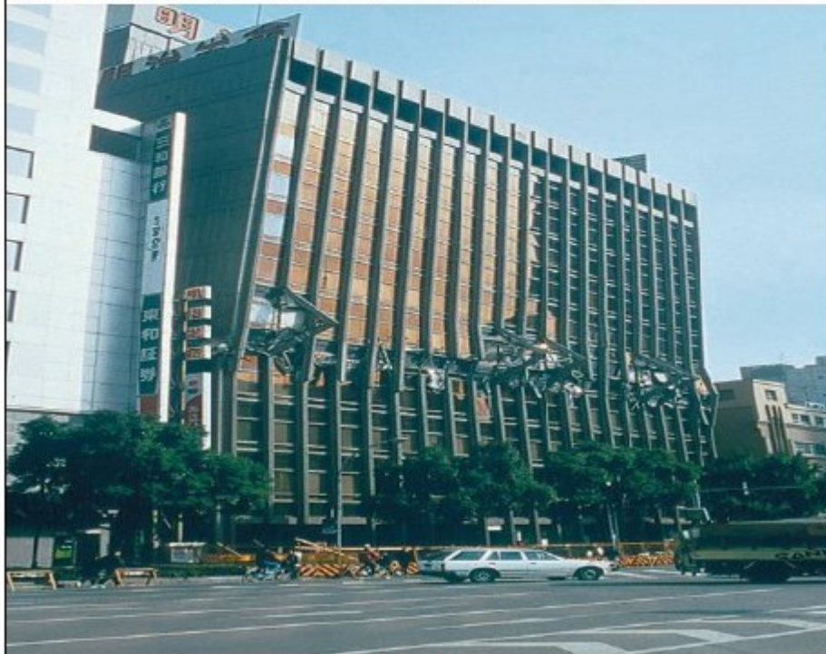
Soft Storey Failure
