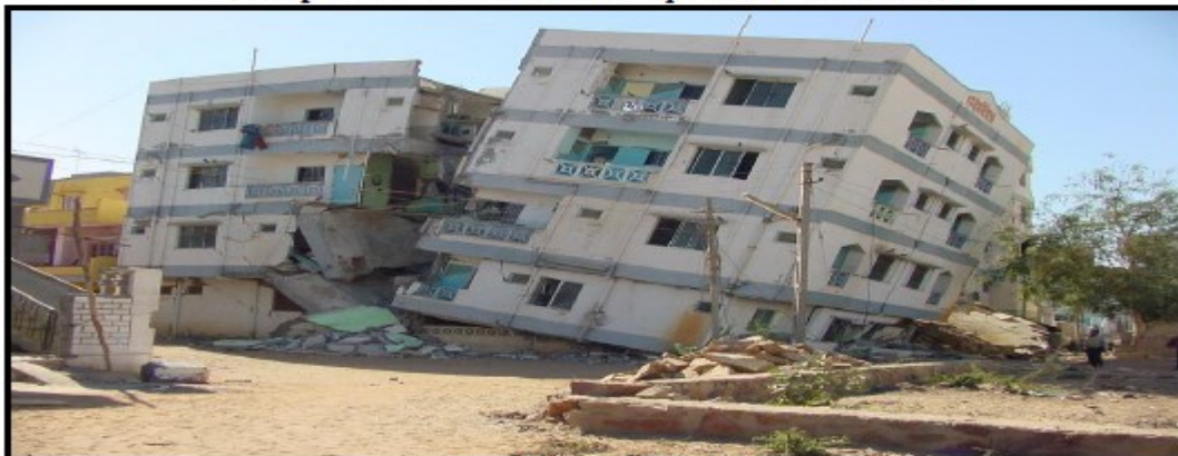
Collapsing a building
