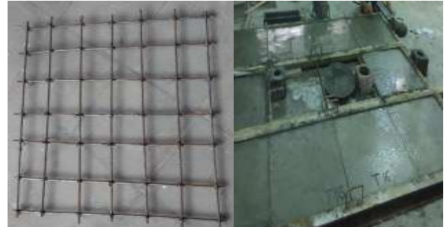
Fig 5: Reinforcement details and slab casting
