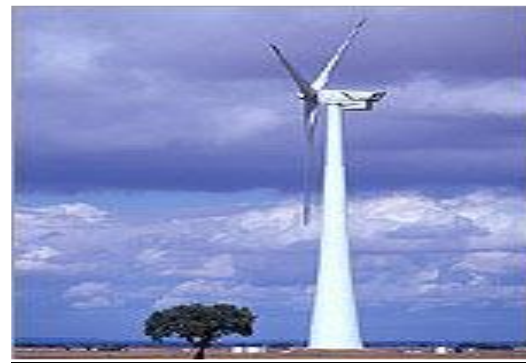
Figure 1.0. GE Wind Energy's 3.6 Megawatt HAWT.
