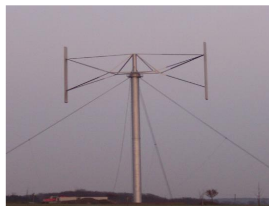
Figure 1.2. An H-Darrius rotor VAWT.
