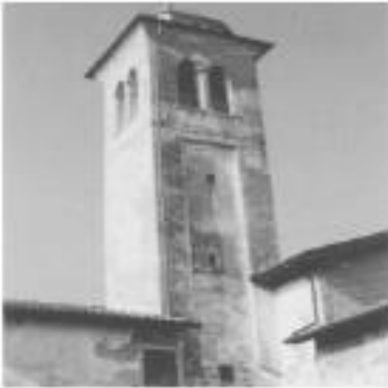
Fig 7: Retrofitting of the bell tower of the Church of San Giorgio at Trignano, Italy
