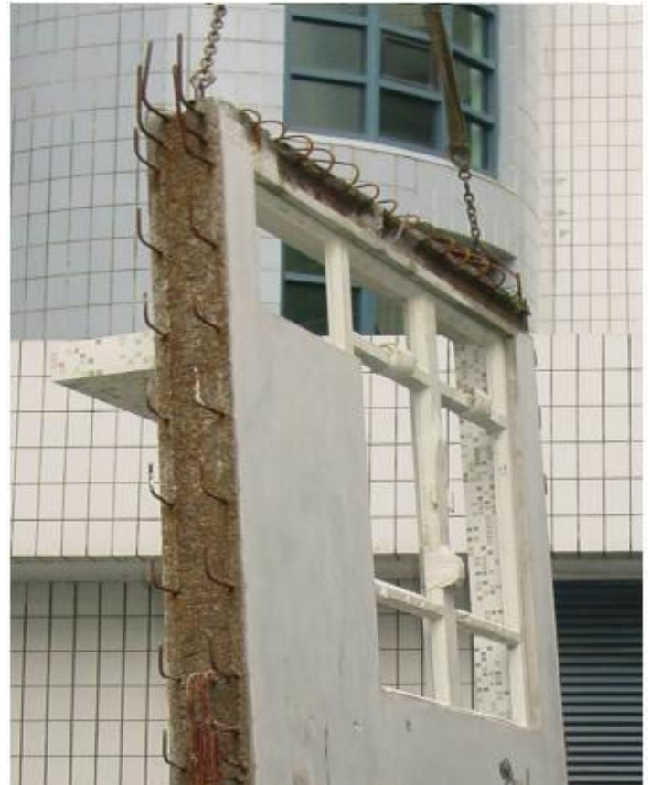
Figure 4: Protocol of finished lightweight concrete precast facade
