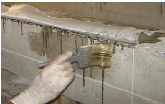
Fig. 3.10 Application of epoxy and hardener on the beam
