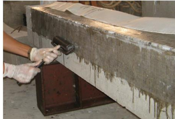
Fig. 3.12 Roller used for removal of air bubbles
