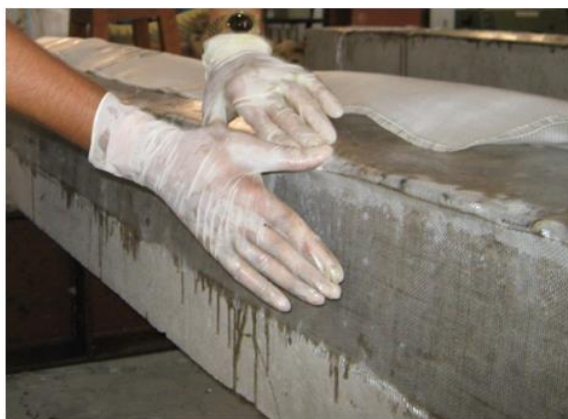
Fig. 3.10 Application of epoxy and hardener on the beam
