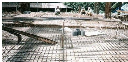
Fig:20: Prefabricated Welded Mesh Less No. Of Workers –Less Construction Cost
