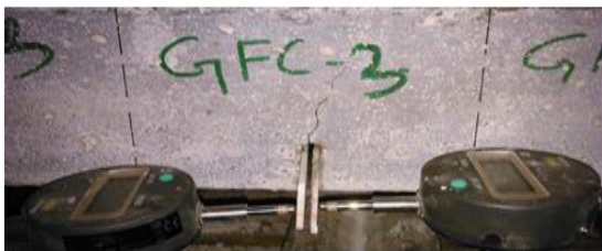
Fig 4.6.5 Crack Pattern of GFC-3
