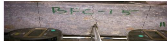
Fig. 4.6.8 Crack Pattern of BFC-1.5
