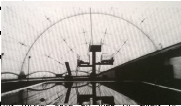
Fig 4 : Internal View of Swimming pool showing double layered membrane roof[barrel form].(3)
