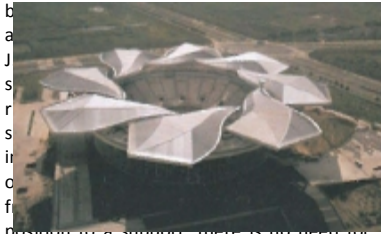
Fig 16: BUILT DESIGN of Qi Zhong Tennis centre, Shanghai Petal form of retractable roof(5)
