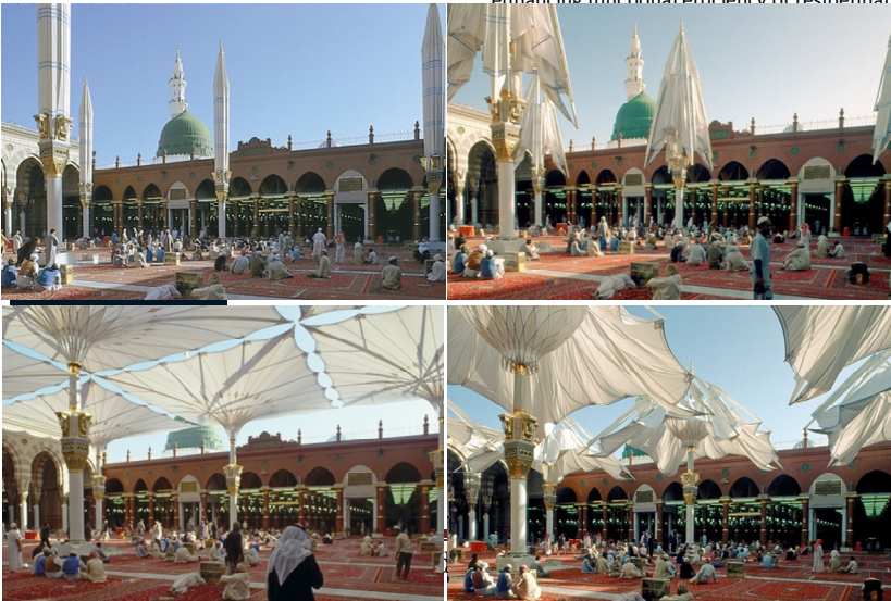
Fig 5: Closed to open position showing folding action of the umbrellas[clockwise from top left]
