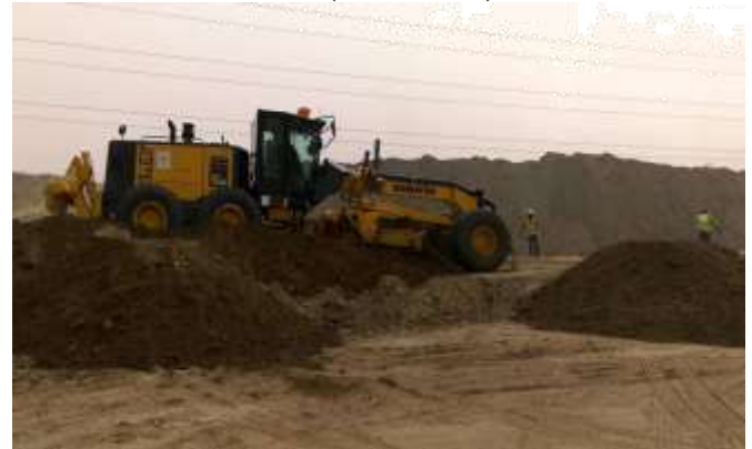
Fig 9: Embankment Filling
