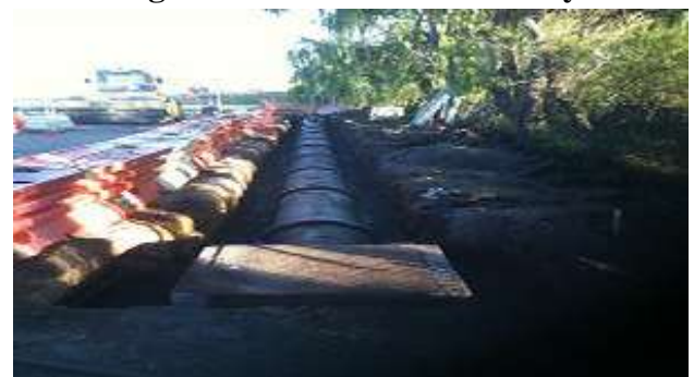
Fig.7: Excavation for Drains
