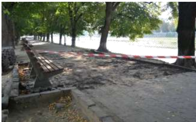
Fig.3: Dismantling of Pavements
