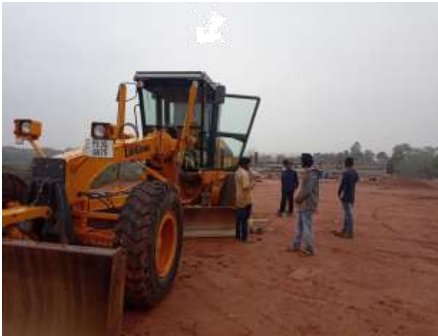
Fig 10: Earthwork for Embankment and Sub-Grade to be placed Against Sloping Ground
