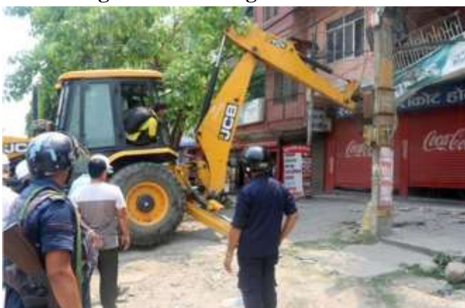
Fig.4: Dismantling of Other Structures
