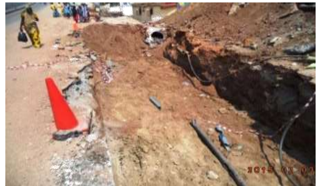
Fig.6: Excavation for Roadway
