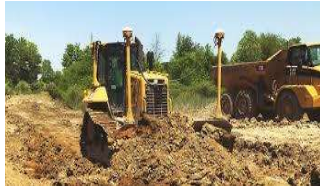
Fig.5: Back filling
