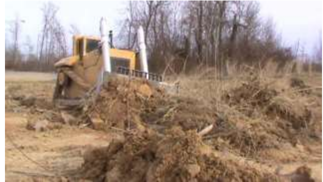
Fig.1: Clearing and Grubbing
