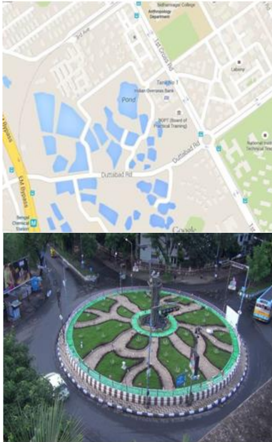
Fig 4.5. Roundabout at Salt Lake, Kolkata
