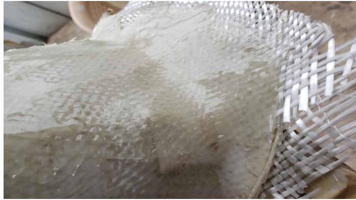
Fig Images after application of resign on fiber
