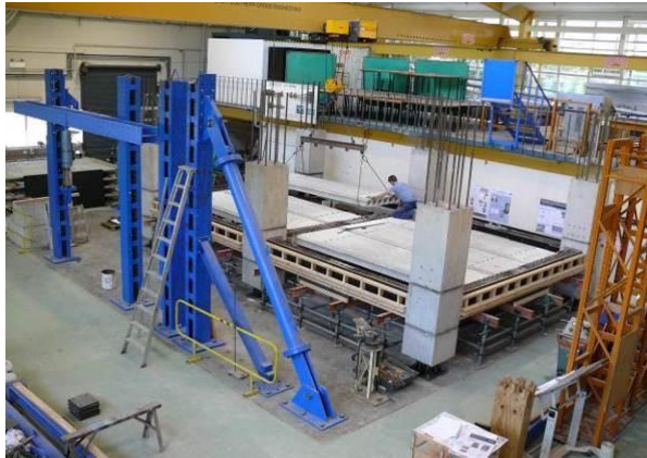
First floor precast components set out
