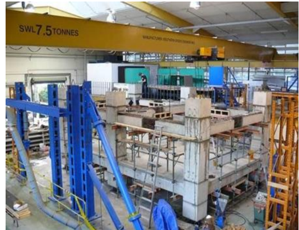
Second floor precast components being grouted.
