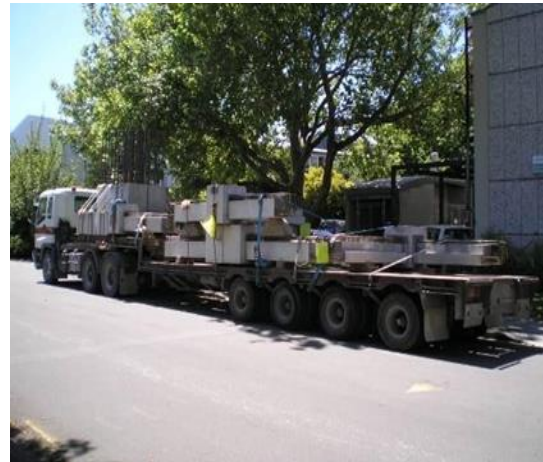
Level one precast components arriving outside laboratory.
