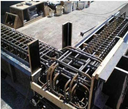
Reinforcement cage in form prior to concrete pour
