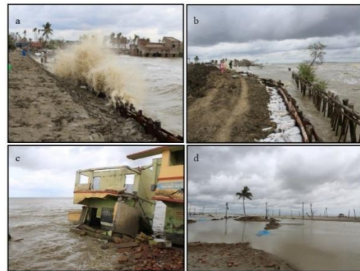
Plate 1. Coastal Erosion in Sagar Island- a: Incoming of high energy waves; b: Breached embankment near Boatkhali; c: Destruction of a school building due to coastal erosion; d: Degradation of mangroves and other vegetation.
