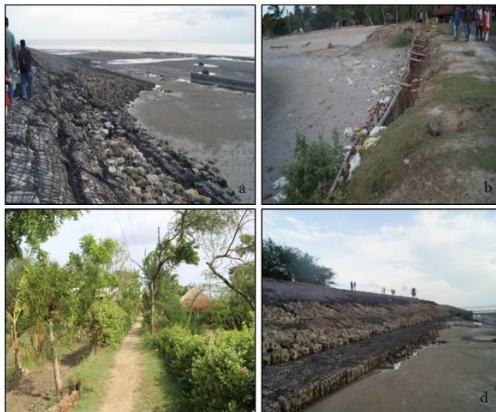
Plate 2. Some suggested measures- a: Net Fencing; b: Revetment; c: Afforestation; d: Sea Wall
