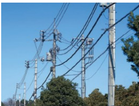
Figure 1: Distribution of overhead cables installing pylons
