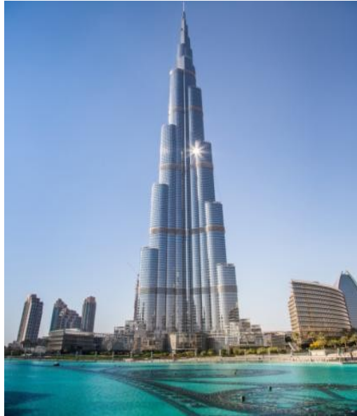
Figure 9: The Burj Khalifa in Dubai is currently the tallest building in the world where the silica fume concrete contributed to record pumping heights of over 600m in a single operation.
