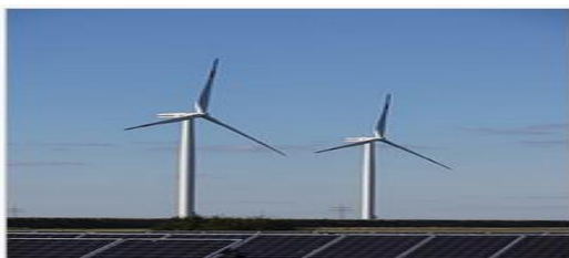
Wind power generation
