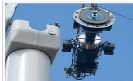
Typical components of a wind turbine (gearbox, rotor shaft and brake assembly) being lifted into position
