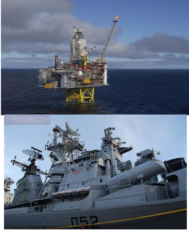
Fig : Gas turbine in offshore service
