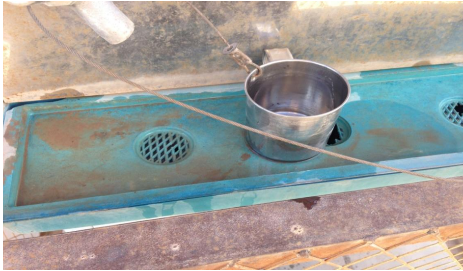
Fig. (3). A steel cup held by steel rope. Rust could be seen in the vicinity of the drinking zone.
