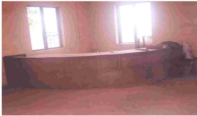
Fig. 1: The Public Library in Ifetedo. It is unkempt and in a state of disrepair.
