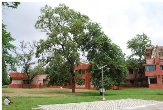
Figure 6. Roof shaded by bamboo trellis and green cover been incorporated in the HVAC design to reduce
