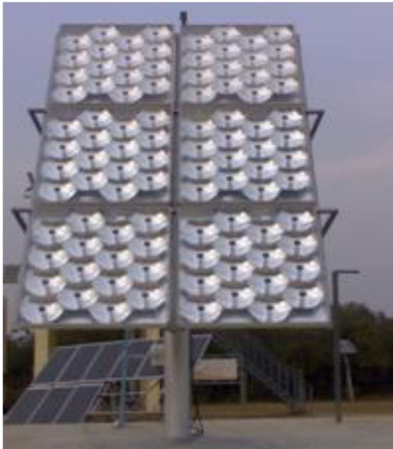
Figure 3. 1.2 KWp High Efficiency Solar Concentrator with Tracker being installed at IIT Kanpur Courtesy: Moser Baer Photovoltaic Pvt Ltd.
