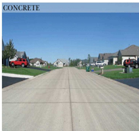
Fig 5. Completed PFRC pavement (ref: http://cebd.asce.org/cgi )
